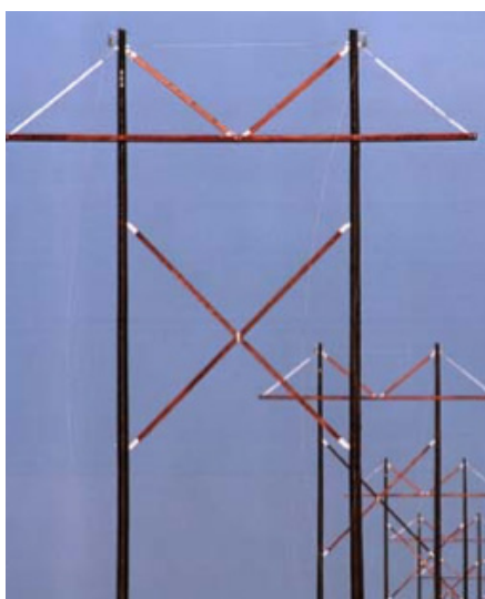
Wood framing up to 345kv
