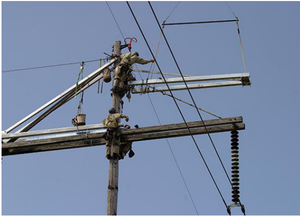
345kv "live" re-framing with Hughes Brothers' steel truss
