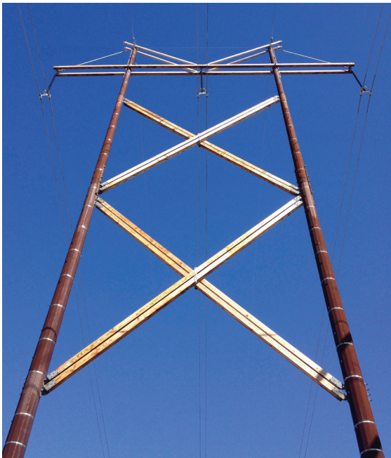
Wood framing on steel poles
