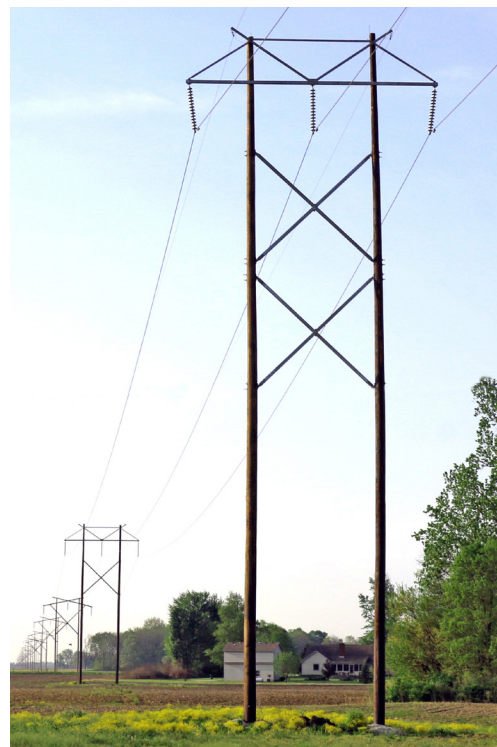
Steel truss on wood poles, shipped pre-assembled for quick installation
